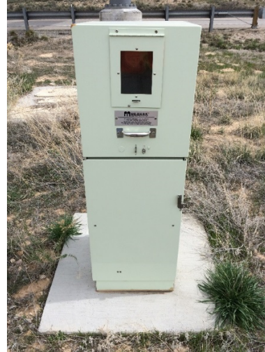
ATMS Power Disconnect Frame - waiting for grounding rod installation
