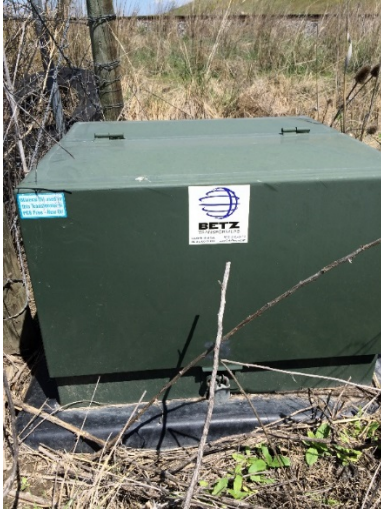
ATMS Power Disconnect Frame - waiting for grounding rod installation
