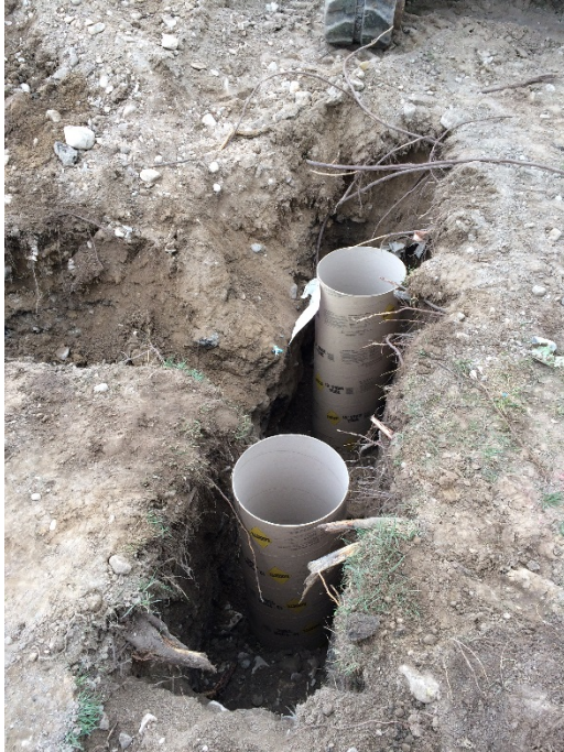
Disconnect Frame – Foundation Forms
