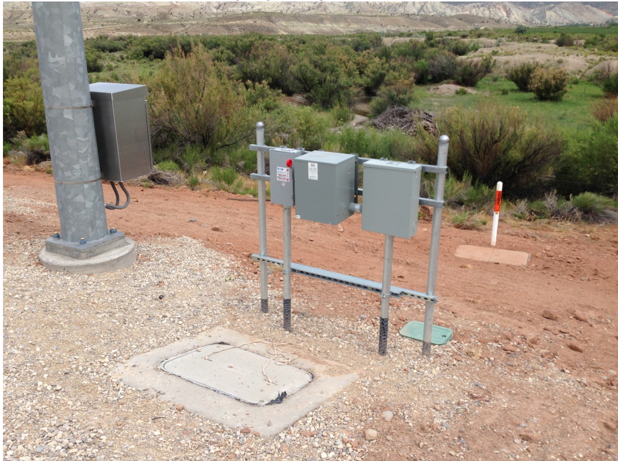
ATMS Power Disconnect Frame - waiting for grounding rod installation
